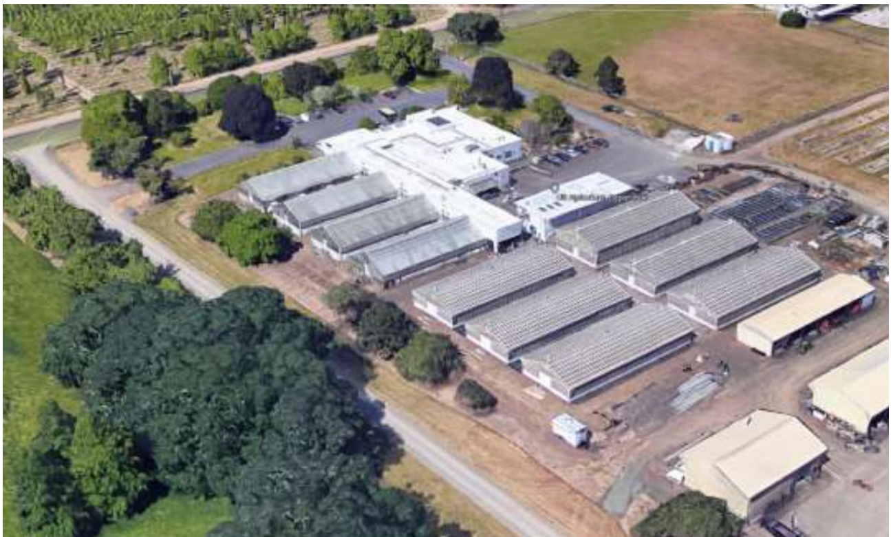
NCGR facilities as of about 2018.
